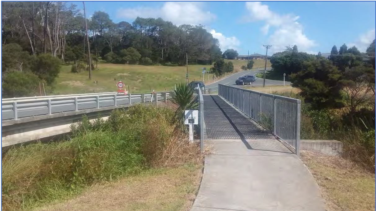
Figure 3: Moir Street Footbridge leading to Tara Road Intersection
